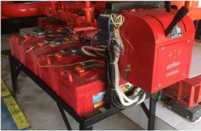
Engine batteries
